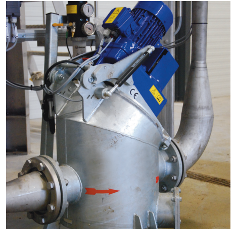
The mixed manure is pumped through a macerator, which ensures that larger particles such as teeth, pieces of wood and the like are grinded so that they do not log the system and cause unnecessary downtime.
