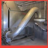
The compression pipe is shaped to ensure optimal transport of compressed screen material to the container.
