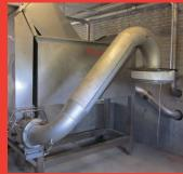
The compression pipe is shaped to ensure optimal transport of compressed screen material to the container.
