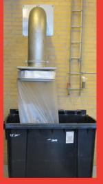
Discharge of compressed screen materials into Longofil bags which are well-suited as disposal bags for screen material. Continuous liner of plastic bags.
