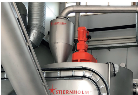
Capacity of the grit washer can be increased by mounting a cyclone at the inlet.
