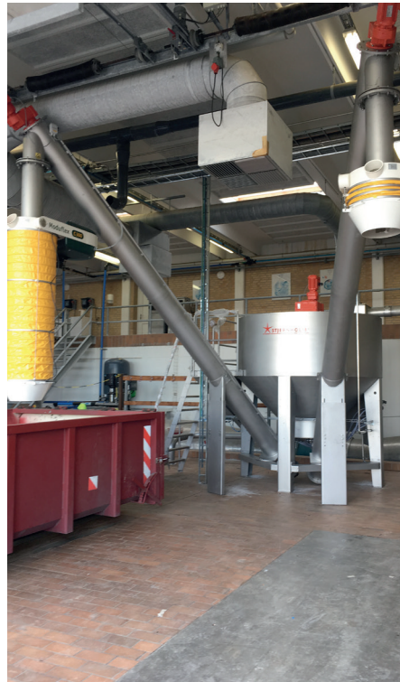
By the addition of a second screw conveyer, the grit output capacity increases to 3 tons/h per grit washer.
