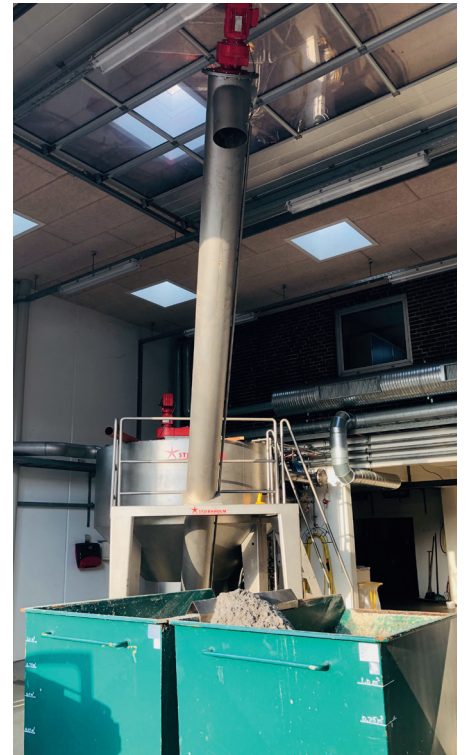
The washed grit is dried by gravity while conveyed directly to a container – ready for transportation and reuse.
