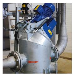
The mixed manure is pumped through a macerator, which ensures that larger particles such as teeth, pieces of wood and the like are grinded so that they do not log the system and cause unnecessary downtime.
