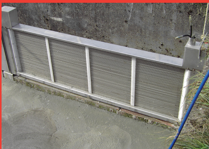
The VR screen is cleaned hydraulically, and consists of a number of parallel horizontal screen bars; every alternate bar is movable. The screen is available with 4 to 10 mm screen spacing, which under normal operation will ensure retention of 90% of the screen material.
