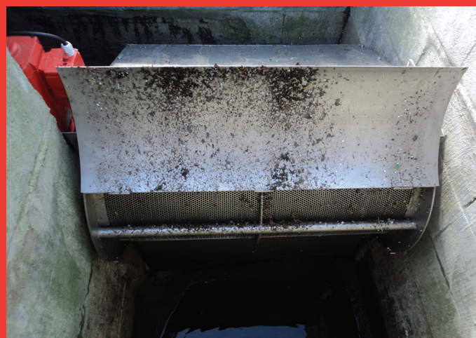
The RO screen is cleaned by an auger with brushes. Here the screen material is retained inside the screen by means of a perforated plate. It is available in three different dimensions and can be supplied with capacity as high as 1200 litres per second.
