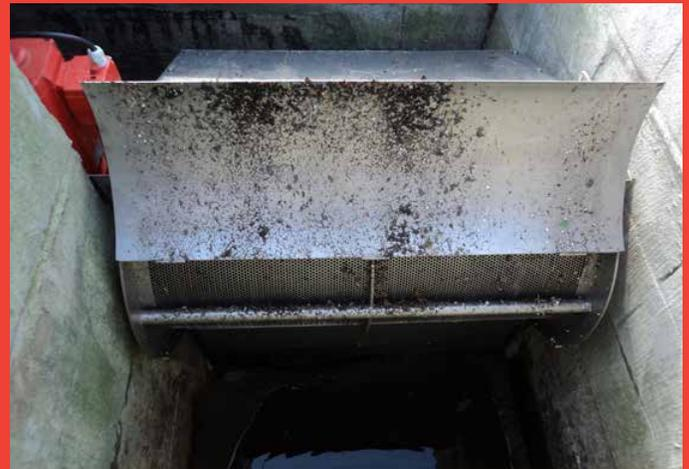
The VR screen is cleaned hydraulically, and consists of a number of parallel horizontal screen bars; every alternate bar is movable. The screen is available with 4.5 mm or 10 mm screen spacing, which under normal operation will ensure retention of 90% of the screen material.
