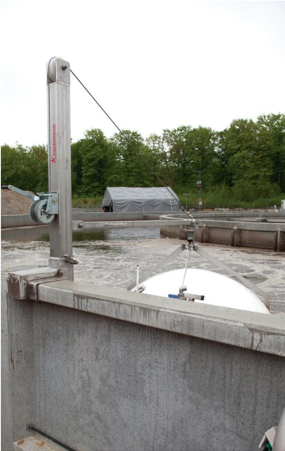
*The bracket makes it possible to raise and lower the unit, turn it 360 degrees and lock it in any position. This makes inspection and service easier.*
