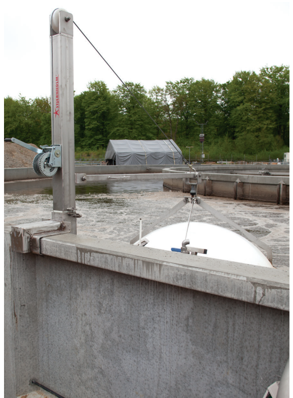
The bracket makes it possible to raise and lower the unit, turn it 360 degrees and lock it in any position. This makes inspection and service easier.
