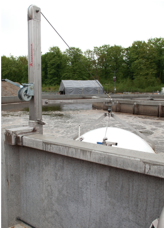
The bracket makes it possible to raise and lower the unit, turn it 360 degrees and lock it in any position. This makes inspection and service easier.
